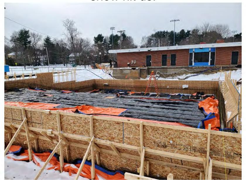
Out front the team built an enclosure and provided temp heat to form and pour the new fully accessible ramps.
