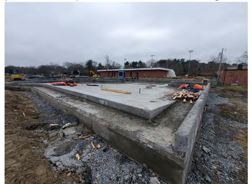
With the new competition pool poured, the team got to work forming the new fully accessible ramp.
