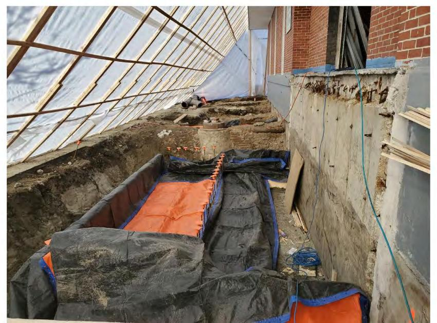
Once the pools were formed, crews installed the wire mesh to prepare for our first concrete pour.
